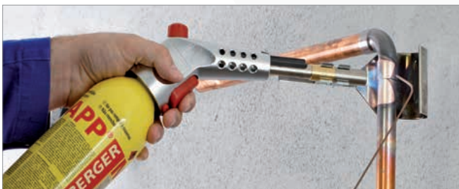
Brazing in gas installation
