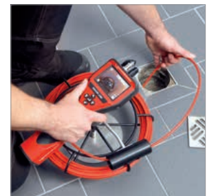
Inspection of floor drains
