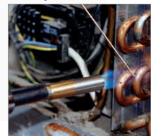
Brazing in aircon and refrigeration
