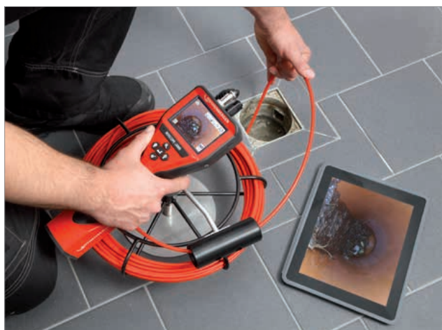
Inspection of basin drains
