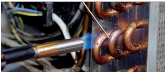
Brazing in aircon and refrigeration
