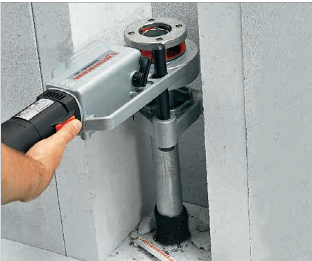
Work in confined spaces
