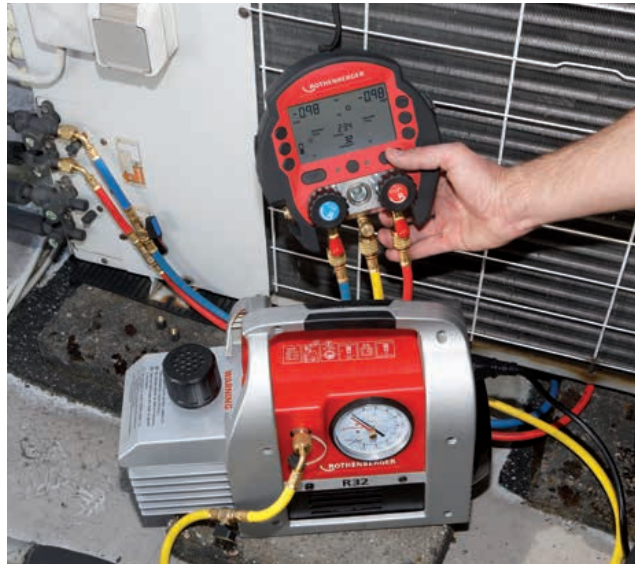
ROAIRVAC - vacuum pump in use with the digital manifold ROCOOL 600
